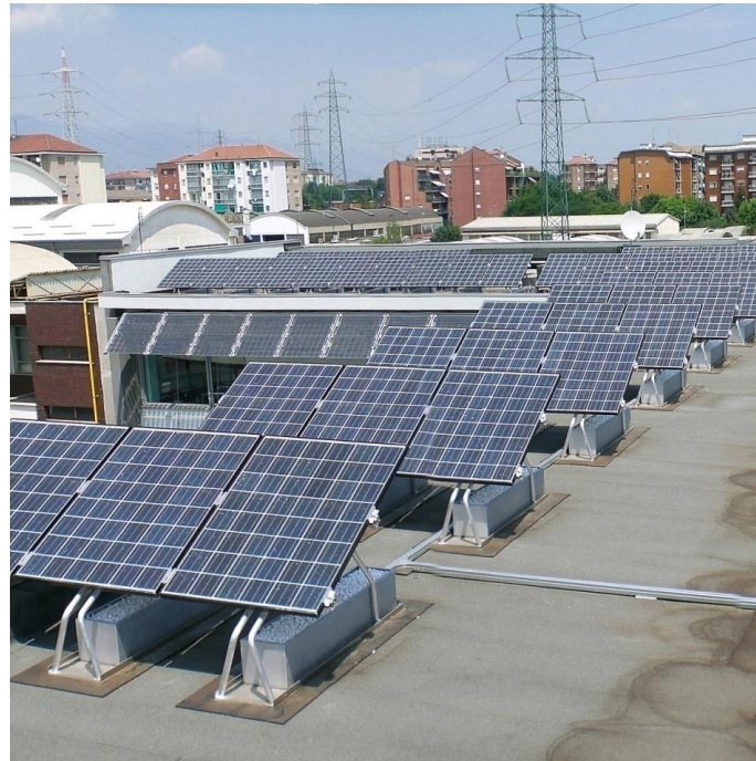
Roof mounted PV system | Rivoli (To – Italy)
