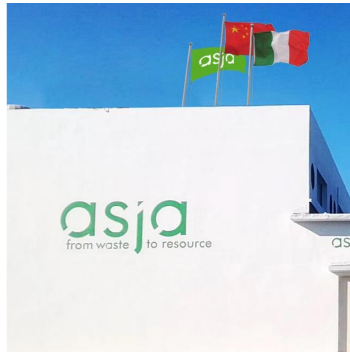
Landfill gas plant | Shenyang (China)
