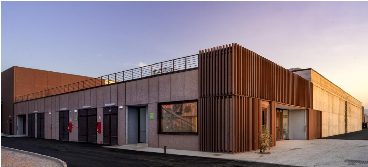
Biomethane production plant from OFMSW (Foligno, Pg - Italy)
