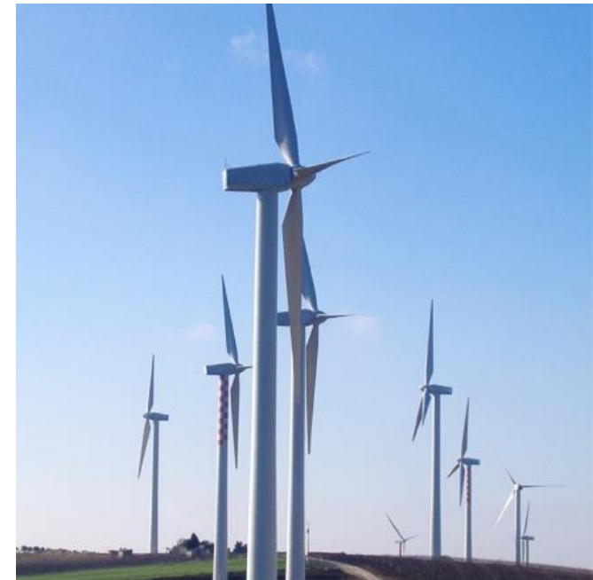
Wind farm | Fumosa (Tp, Italy)
