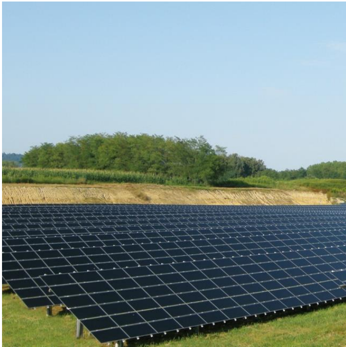
PV plant | San Giorgio (To - Italy)
