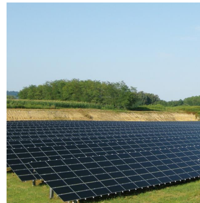
Planta FV | San Giorgio (To - Italy)
