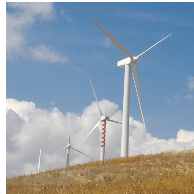
Parque Eólico | Guarine (Tp, Italy)
